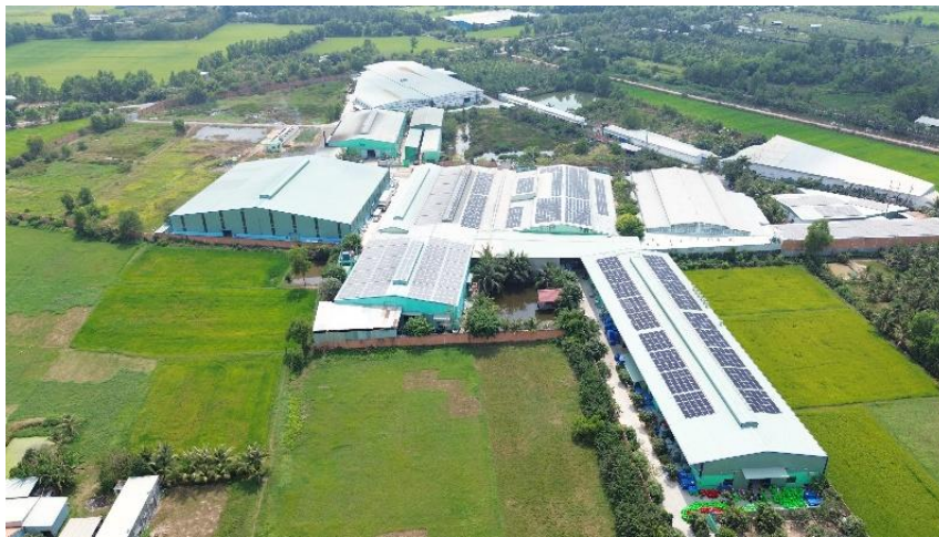
Figure 5. Installed 200 kWp Solar System
