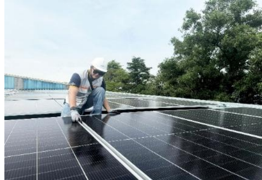
Figure 2. Stride conduct the QA steps at one roof top solar project
