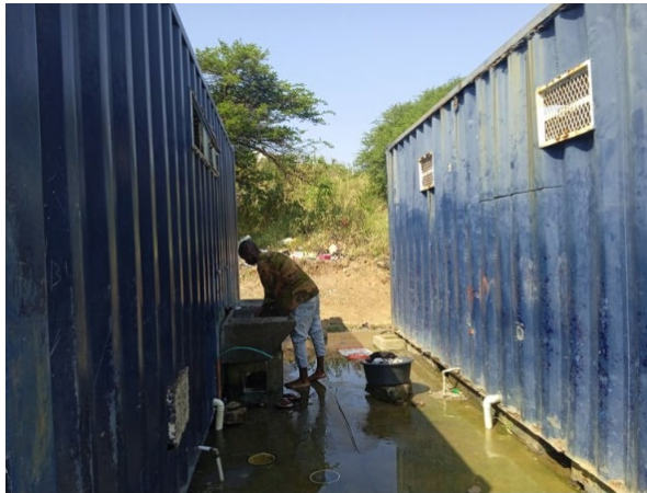
Figure 1. The state of community ablution blocks in eThekweni Municipality
